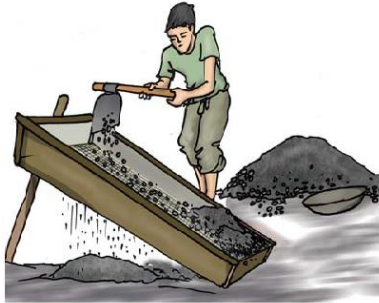
4. Pebbles and stones are removed from sand by sieving.
